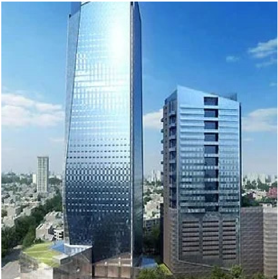
Transformation of Mill Land into High-Rises
