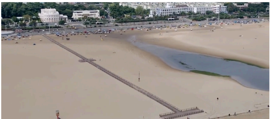
Pathway for persons with disability at Marina Beach, Picture Credits: Greater Chennai Corporation
