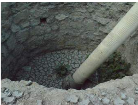
Figure 2-17: Tube pulled out of percolation well at Bodakdev
