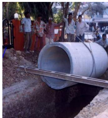
Figure 2-2: Sewerage network being laid near Vastrapur Lake
