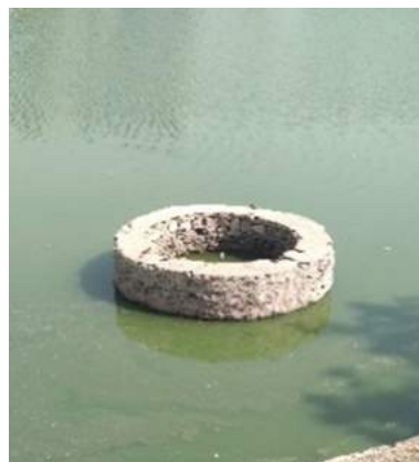
Figure A-6: Percolation Wells at Vastrapur Lake
