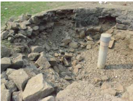
Figure 2-16: Damaged Percolation well at Ranip
