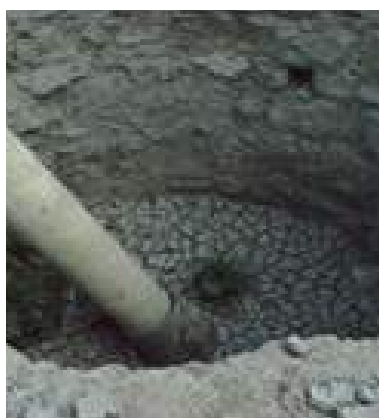
Figure A-34: Damaged percolation well
